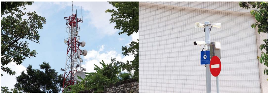
Figure 8 High Ground Alarms and Loud Speakers in Macao SAR. a) One High Ground Alarms located at the high hill of Macau Peninsula. b) Loud Speaker on a pole.
